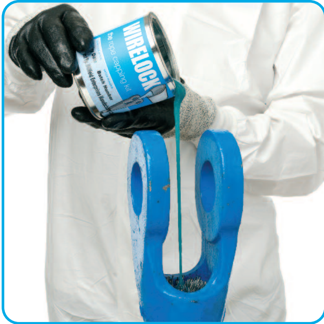
Figure 9: Upon mixing the compound should be poured immediately.
