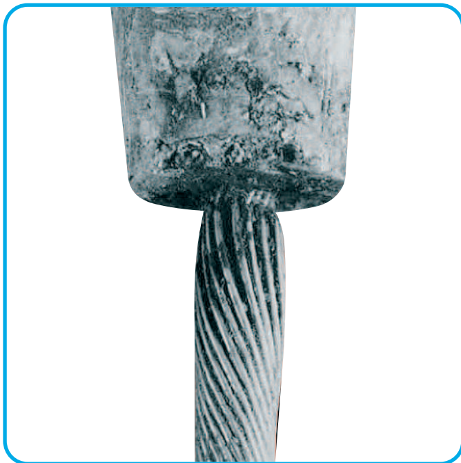
Figure 11: Typical example of the swelling of stainless steel rope due to Crevice Corrosion
